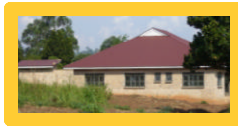
The new Miriam Duggan Home under construction
